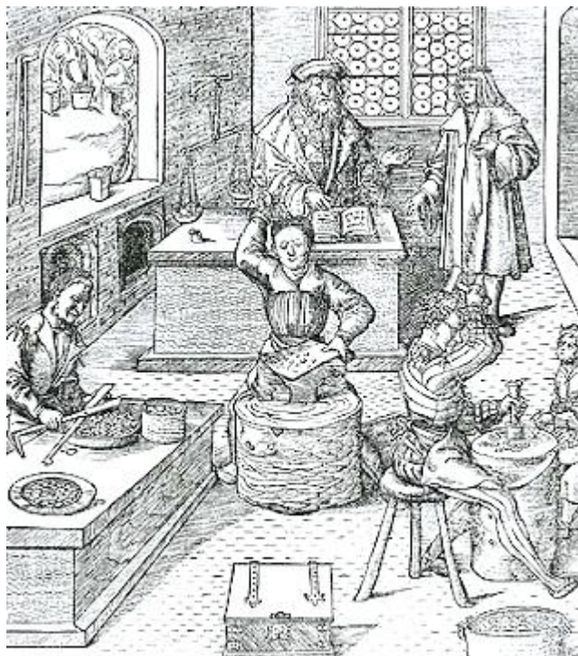
Figure 2.13 – Hans Burgkmair the Older and Leonhard Beck, Maximilian at the Mint in Hall-in-Tirol , 1510. On the left is a furnace for smelting the metal. In the centre, the metal is being hammered into a sheet (in reality this would have been a strip rather than a rectangle). In the front left, coin blanks are being cut. In the front right, the coins are being struck.
