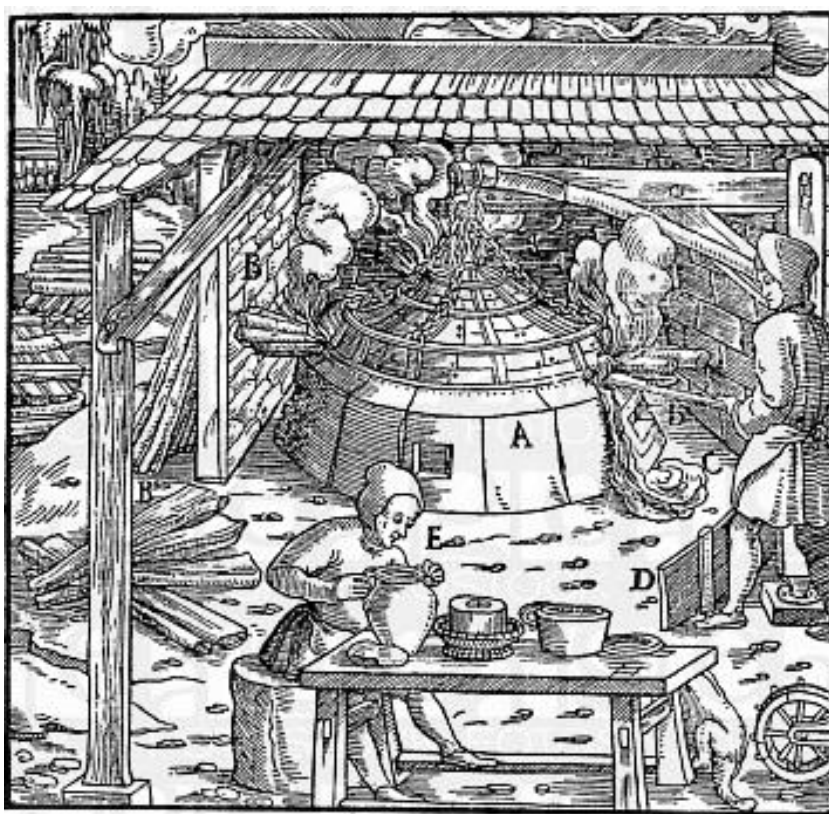
Figure 2.1 - A cupellation furnace with hearth in place. “A – Furnace. B – Sticks of wood. C – Litharge. D – Plate. (E – The foreman when hungry eats butter, that the poison which the crucible exhales may not harm him, for this is a special remedy against that poison.”) (Agricola, 1950 [1556]:474)
